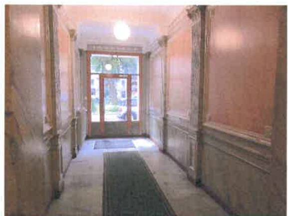
Trapphus i gott skick
